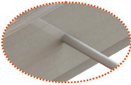
Tie bar fixed to the eaves beam
