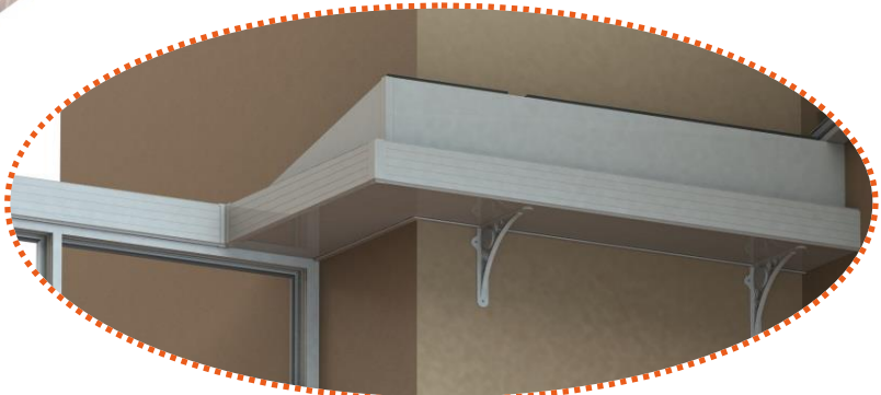
Internal cladding for raised back box gutter. Viewed from below.
