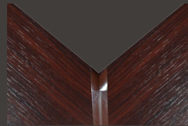
Brown window board angle joint
